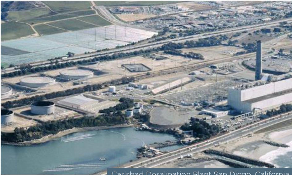
Carlsbad Desalination Plant San Diego, California
